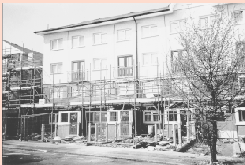
SRB-funded improvements in low-rise flats/maisonettes
